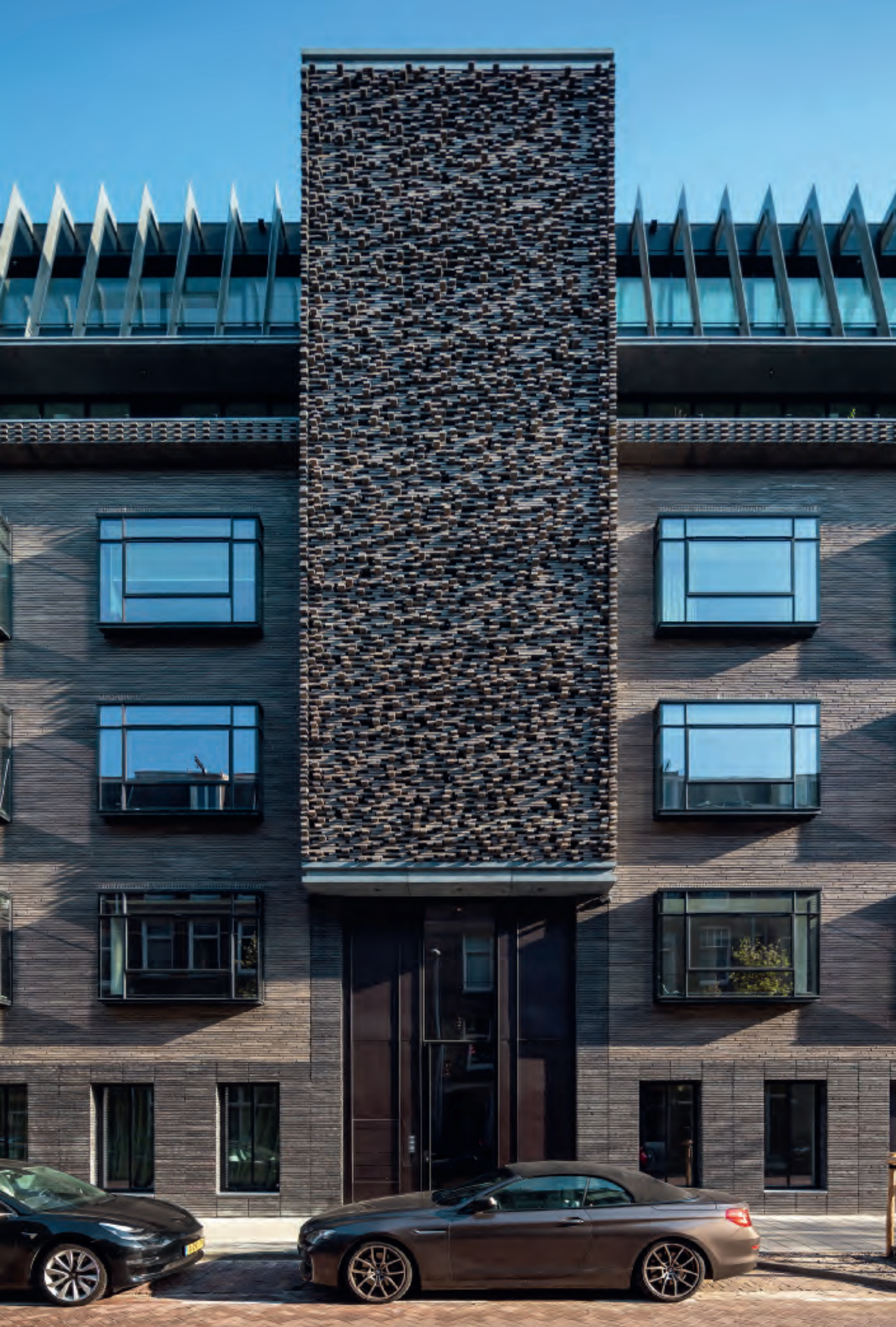
Ruysdaelstraat 77–89 creatively exploits the myriad opportunities afforded by brick. Three different Kolumba bricks and six different bonds have been used, including in the relief pattern in the large frontispiece.
