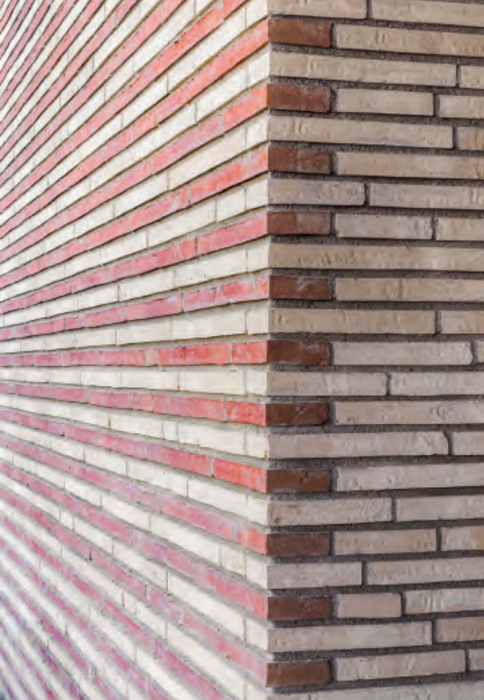
The façade towards the schoolyard uses K71 and K23.
