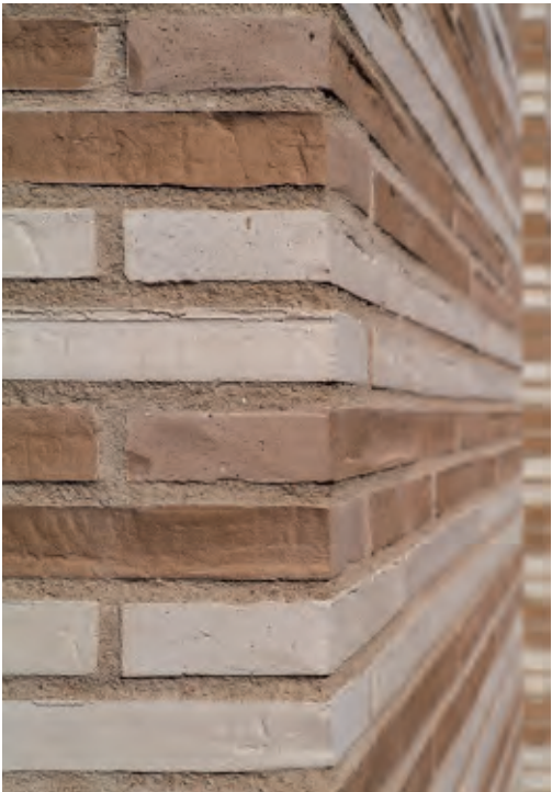
The striped façade is achieved with two x two courses with runner bonds in K11 and K21.
