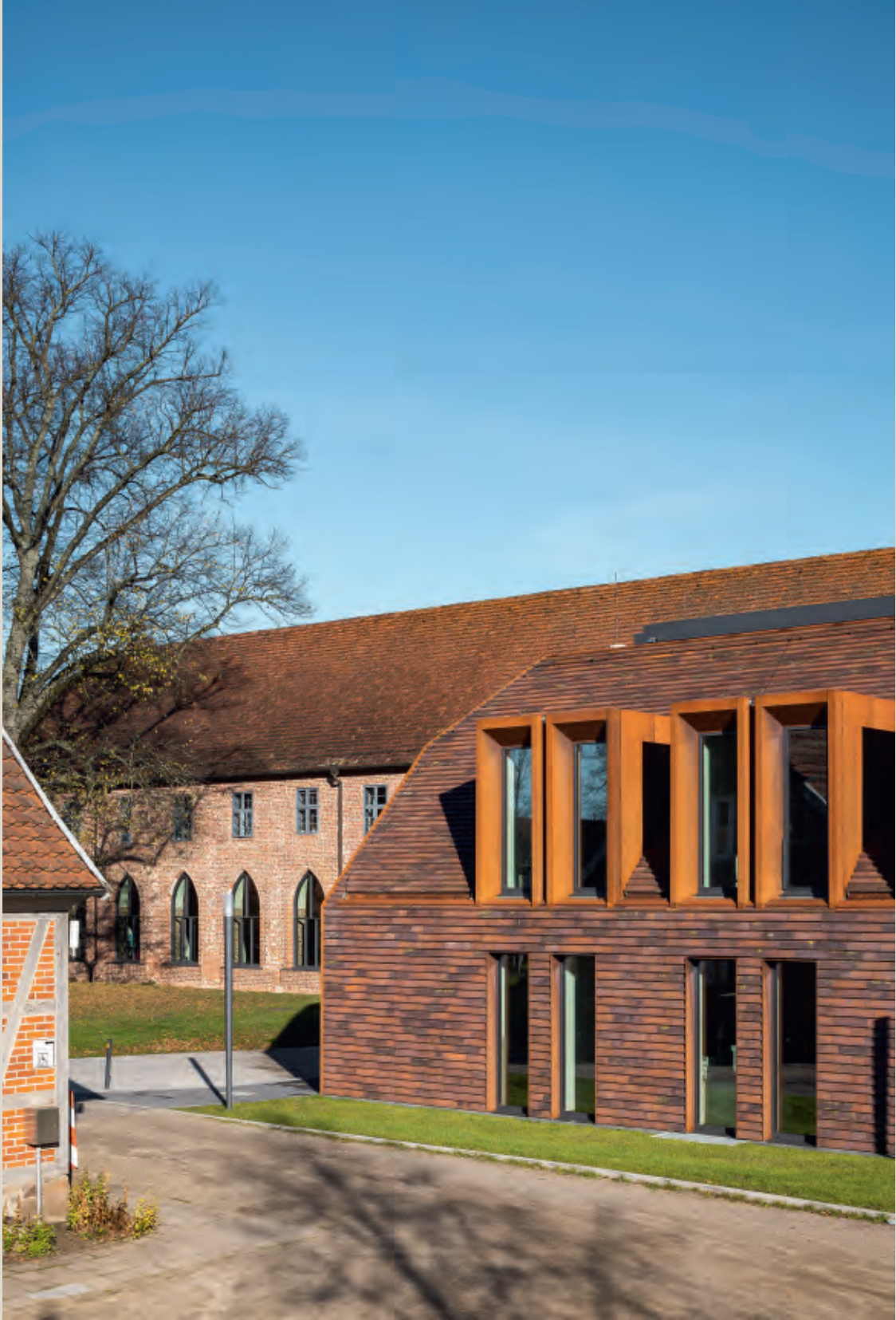
Three-metre-high dormer-style windows provide space and bring plenty of light into the first floor. The dormers and window surrounds are made of Corten steel, in shades that match the tile.
