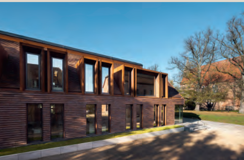
Three-metre-high dormer-style windows provide space and bring plenty of light into the first floor. The dormers and window surrounds are made of Corten steel, in shades that match the tile.
