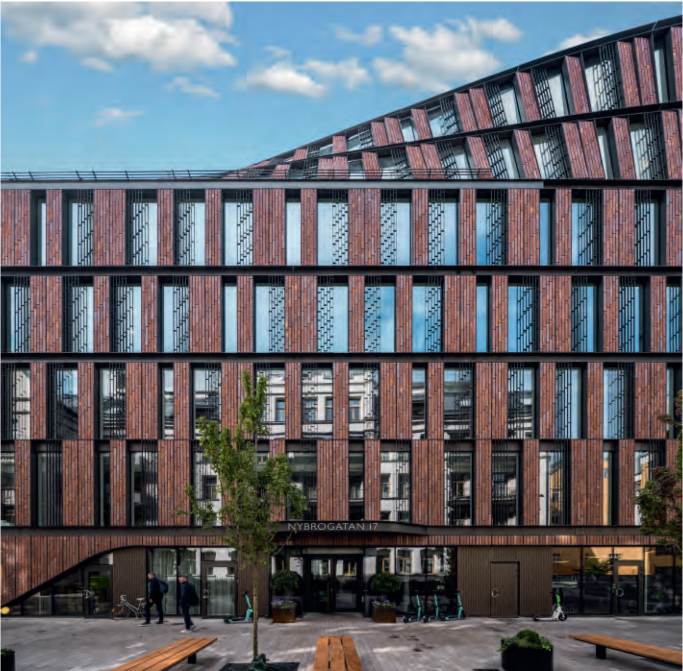
The roof of Astoria House and the façades on the office building are clad with vertical Kolumba in an extra-long format.
