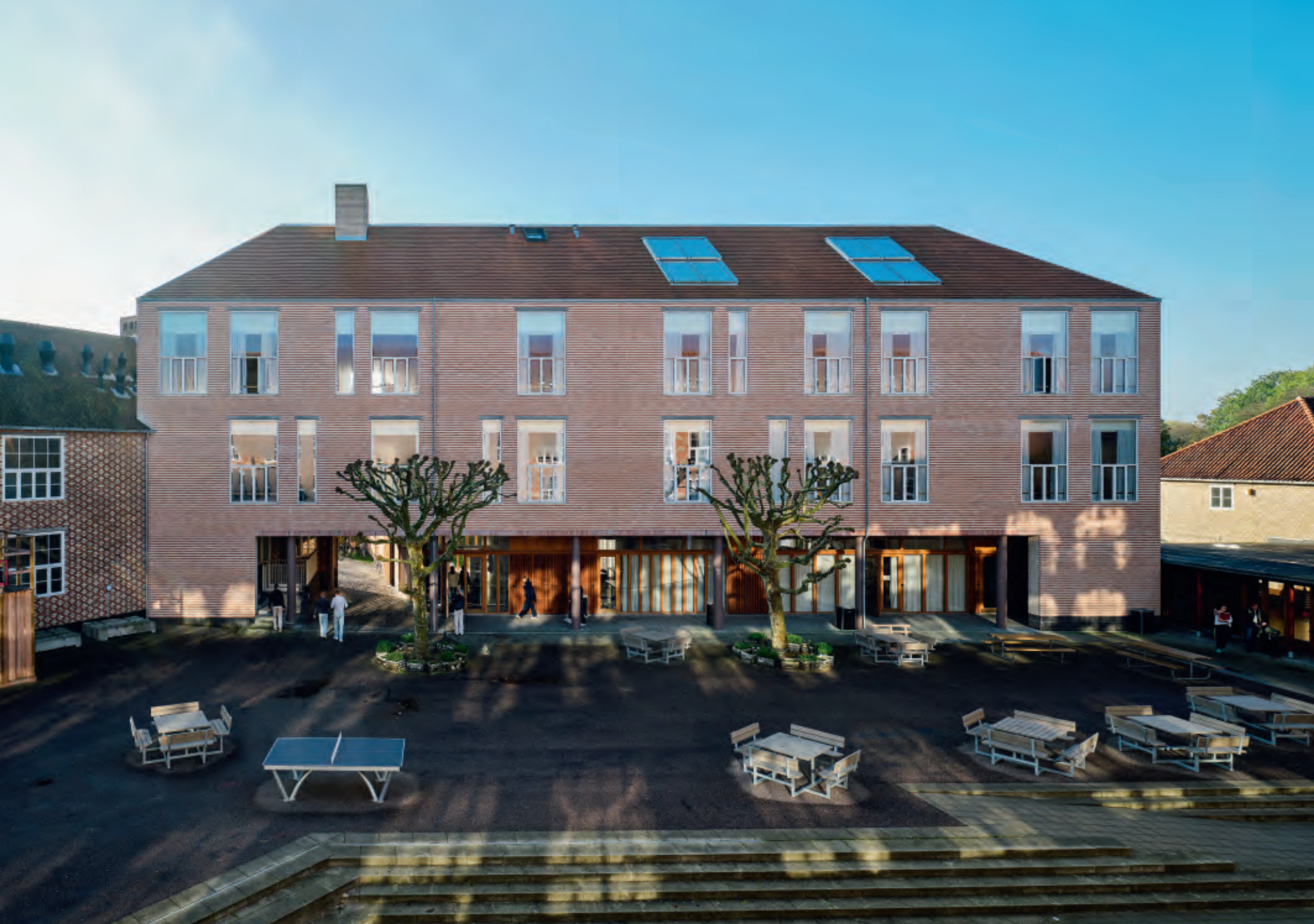
The east gable on the new wing is joined to an existing wing of the school. The west gable is freestanding. All of the façades facing the schoolyard are in yellow and red brick. The patterns on the old façades have diagonal lines, while the new wing has narrow horizontal stripes and a lighter, crisper look.
