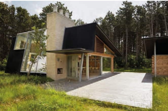
The house is made of pine felled on the site, while the roof is a steel construction.
