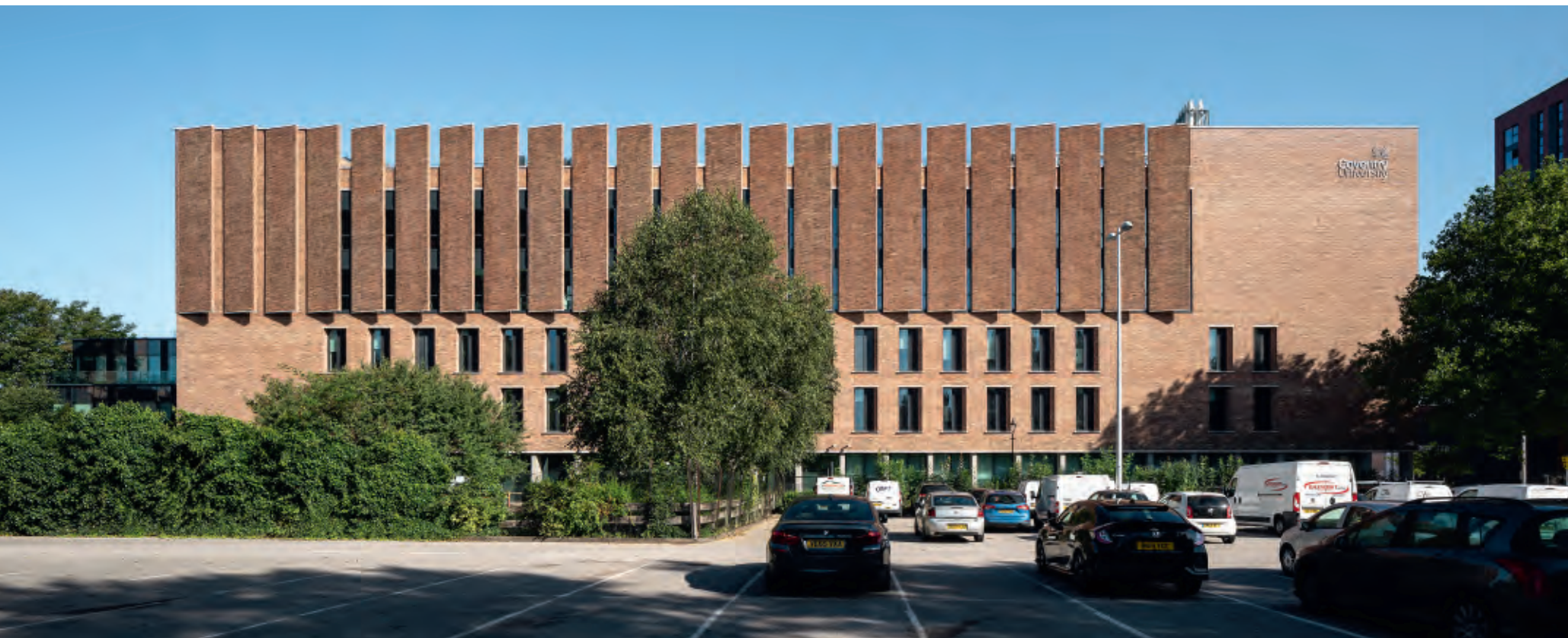
The new campus building's most distinctive feature is its south-facing façade. It is visible from quite some distance and embodies the architects' aim of creating a high-quality landmark building for the university.
