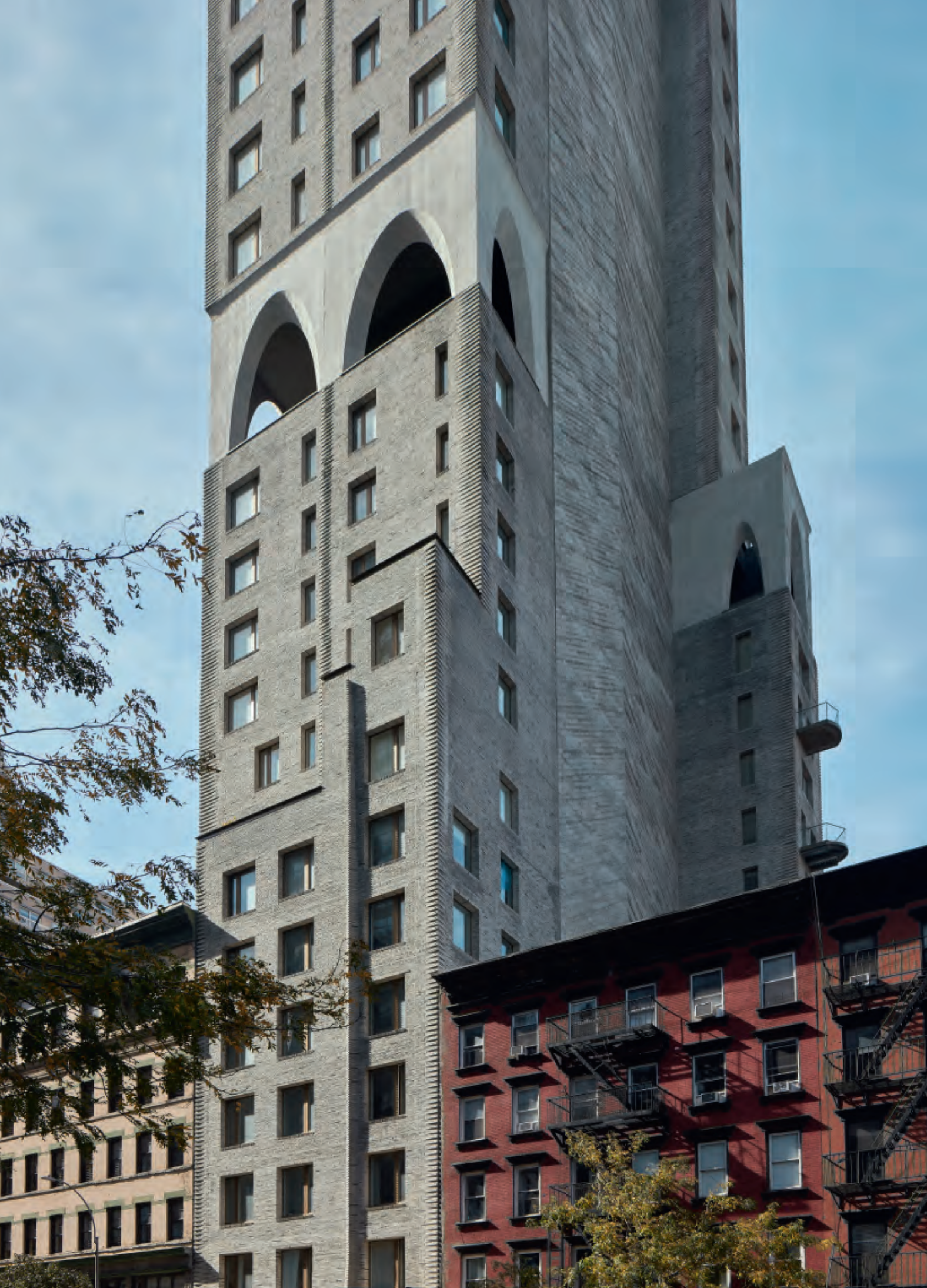
180 East 88th Street is a concrete structure cast in-situ with façades clad with brick on site. A vertical section in full length of the tower on the north side has exposed concrete, as does the belt of in-situ cast, parabolic arches.
