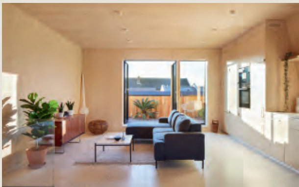
Floors are whitewashed ash or terrazzo tile. Wall and ceilings are exposed Cross Laminated Timber.
