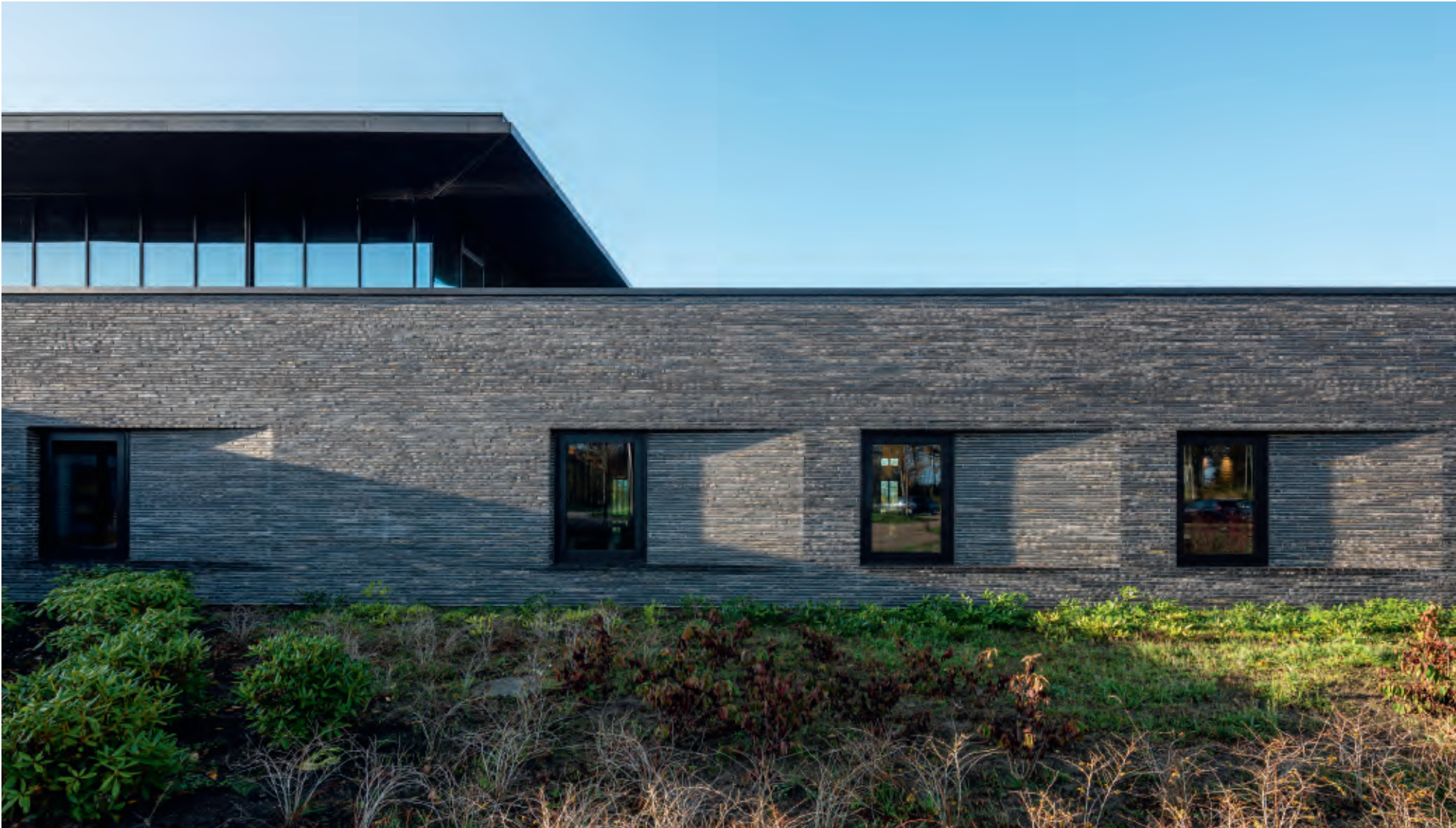
Elongated Kolumba brick in a grey-brown shade reminiscent of bark emphasises the horizontal idiom and brings the building into harmony with the surrounding nature-reserve forest.
