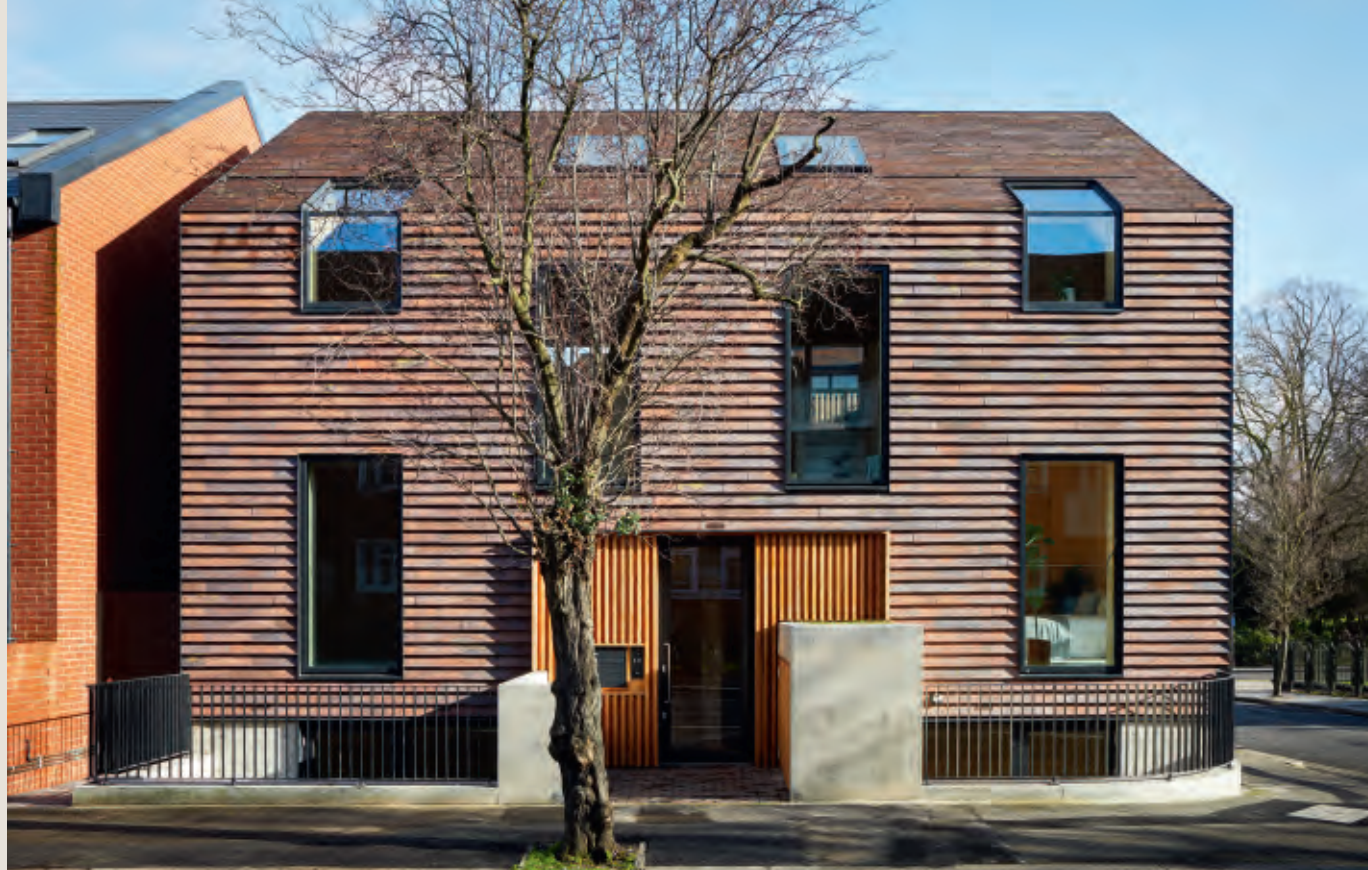
The new complex mimics the surrounding buildings without plagiarising them. The choice of Cover meant the façades and roofs could be treated as a single surface with uniform windows, emphasising the holistic sculptural idiom.
